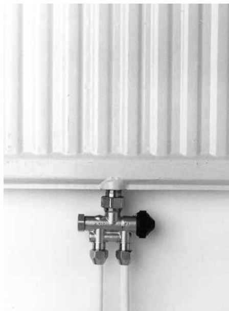
1-strengsventil, undermonteret
